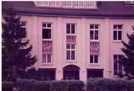
2-28 FA Dining Facility (Mess Hall)
